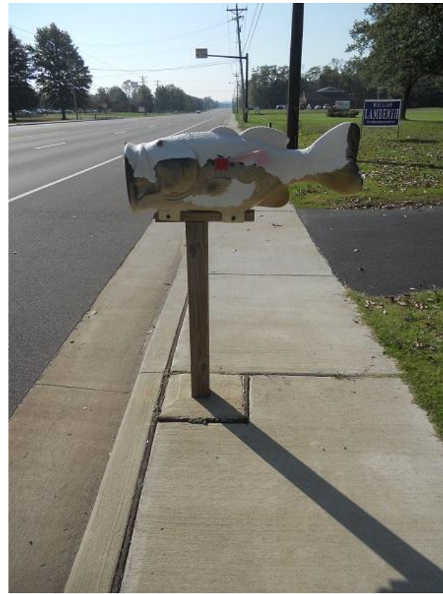
Non-Compliant - More than 4" overhang in "protected zone"
