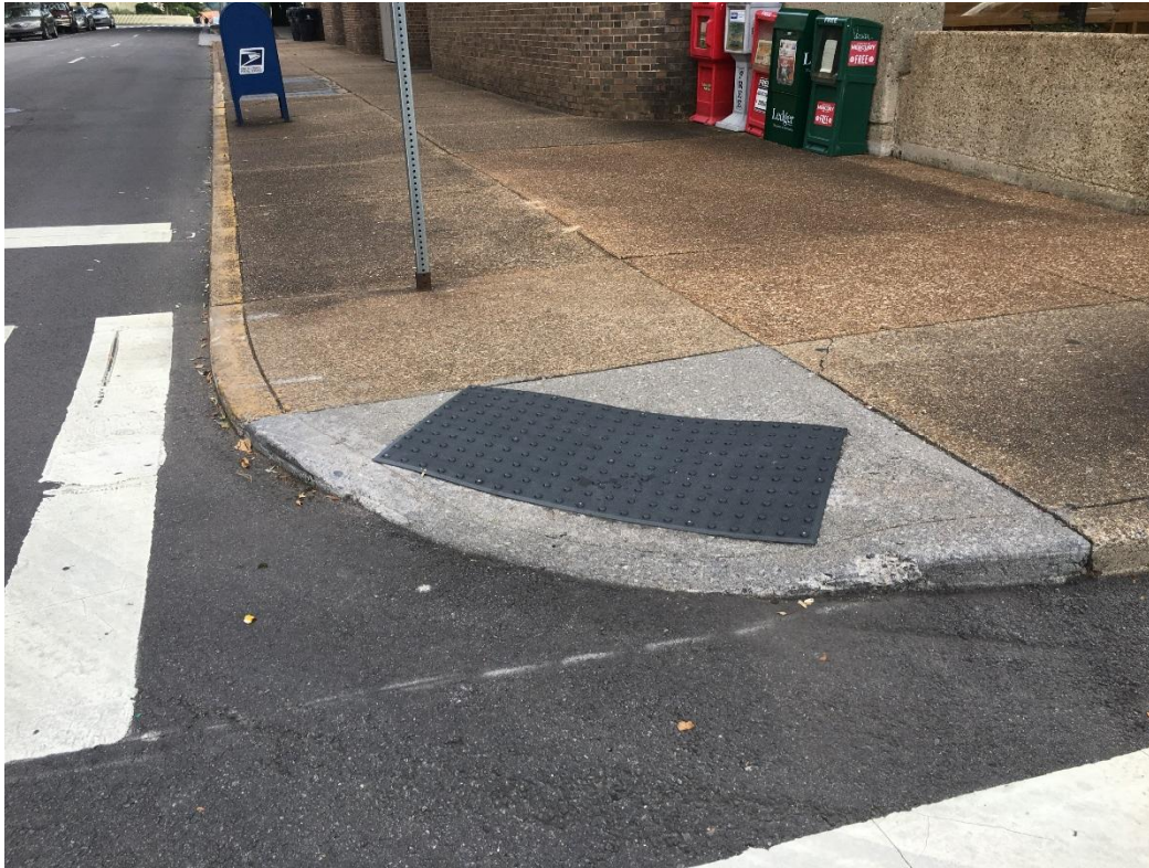
Retrofit installation on non-compliant curb ramp
