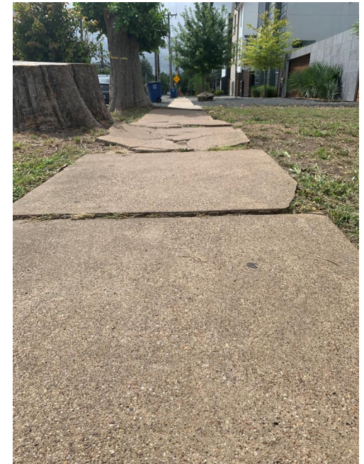
Cracking/Sinking
