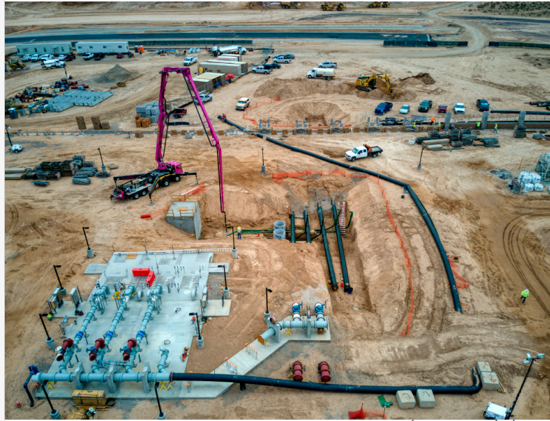
[Caption for Photo Below: Lift Station under Construction]
