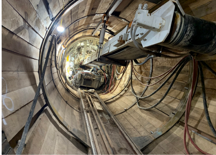
Below: Boring Tunnel in Progress]
